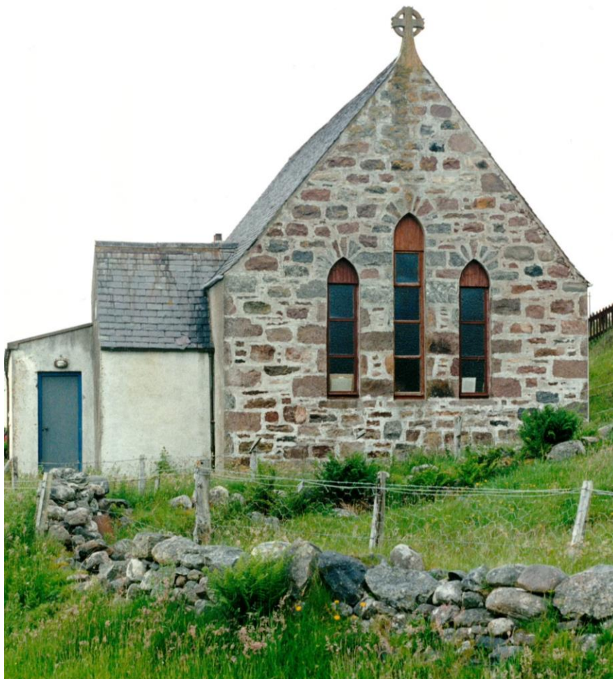
Lodges of the Province – Lodge Lochewe No 1551 - Aultbea
